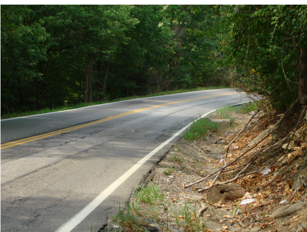
35) KY 1501, Hands Pike Hill looking west at substandard drainage
